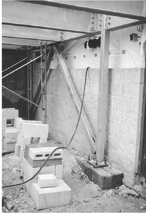
Figure 18-3 Garden hose placed briefly in wall cavity to test for obstruction of water flow to weeps.
